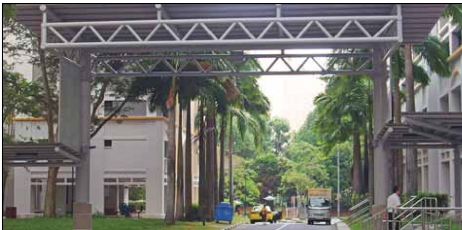
New covered linkway and drop-off porch at Block 946A Hougang Street 91.
