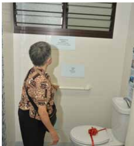
Improvements to the toilets.
